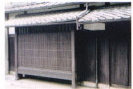
Protruding lattice (degoshi)
